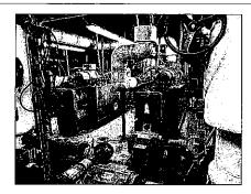
Figure 18: Existing water-cooled screw chillers
