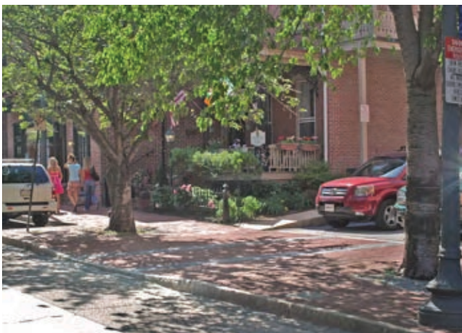
Best Practice example of Brick Crosswalk in Driveway Throat, West Chester, PA
