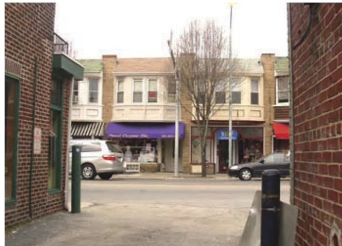
Narrow Curb Cut for Alley in Oakmont Village
