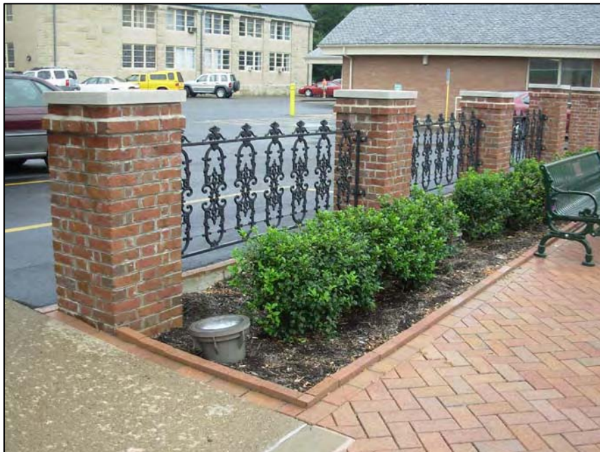
BRICK PIER, FENCE, AND HEDGE AS PARKING LOT SCREEN
