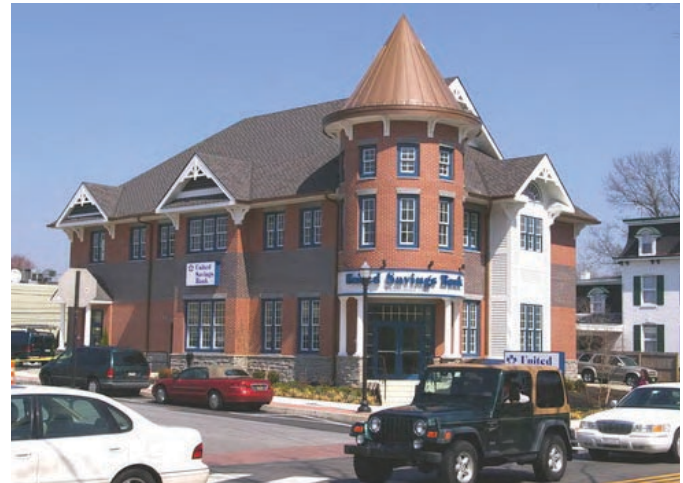
Articulated Facade with Vertical Bays, and Articulated Roof, United Savings Bank, Media, PA
