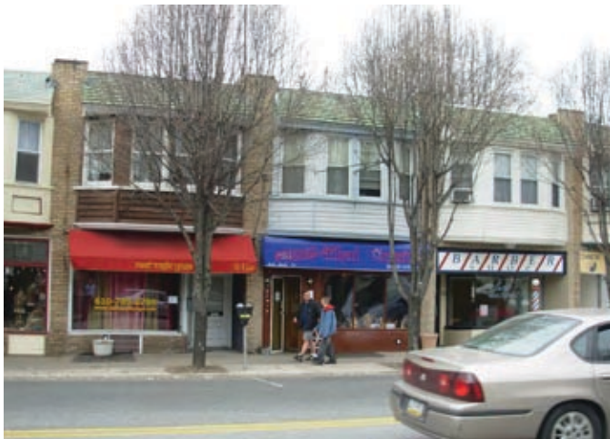
Continuous Curb Without Curb Cut in Oakmont
