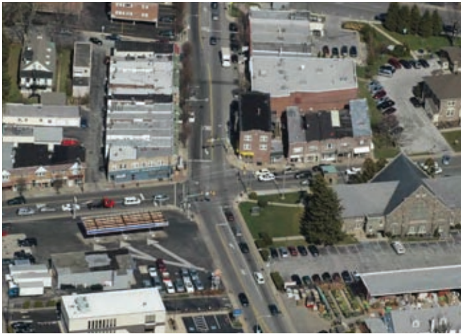
Buildings Located Close to Sidewalks in Oakmont Village and Setback along Eagle Road
