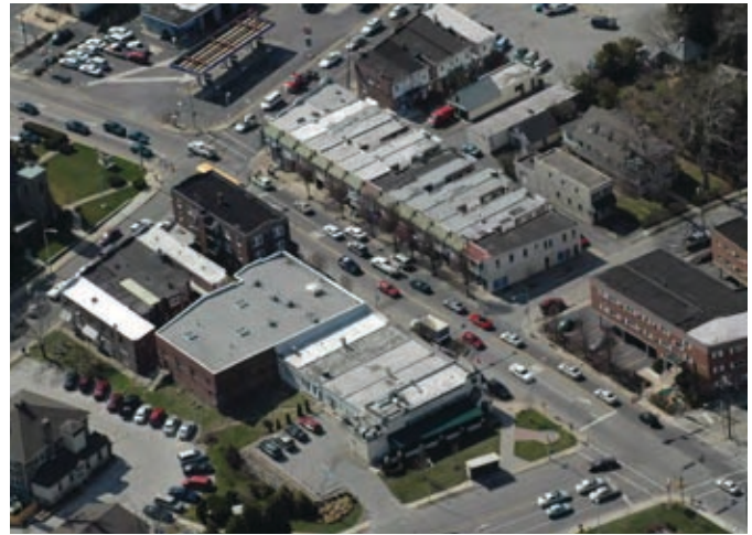
Buildings Grouped Close Together, Oakmont Village
